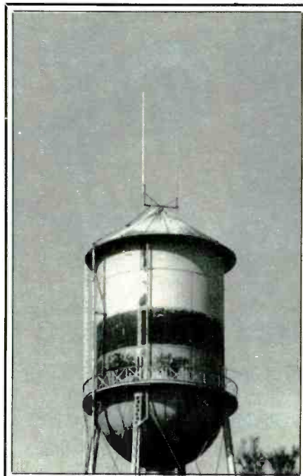
Main Cleveland area repeater antennas cover frequencies 143.99 MHz and 49.49 MHz. This water tank is 174 feet above ground. (Photo by Patrick J. Chick, N8DAQ/AAR5TO)
